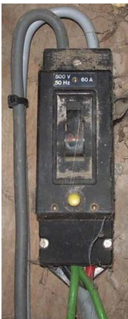
60 A voltage-operated earth-leakage circuit-breaker. Photo courtesy of RF Lighting
