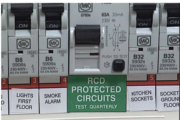
RCD in typical split load consumer unit
